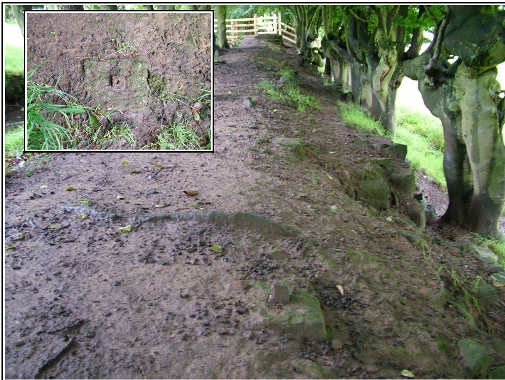
Figure 5. The line of iron railing footings can be seen running along the right side of the path. Inset is detail of a footing.
