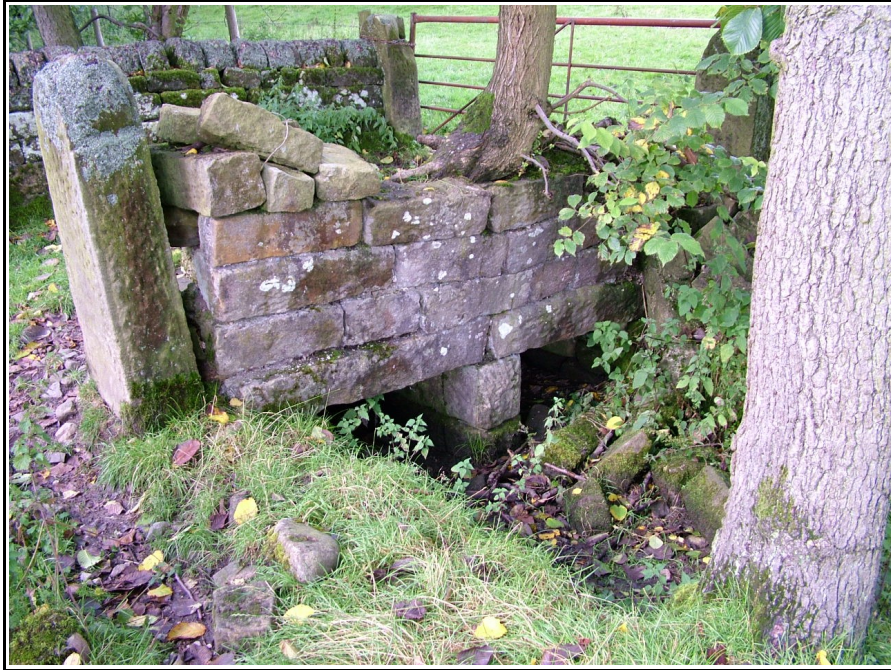
Figure 4. The ornamental bridge over the mill race – note the curved coping stones on the far wall
